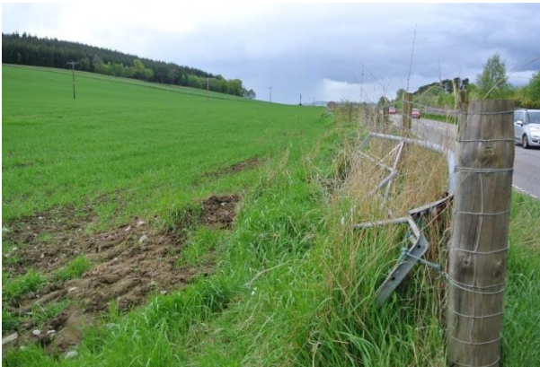
Adjacent to A832 looking west
