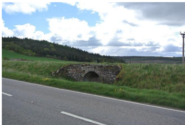
Disused rail line and bridge
