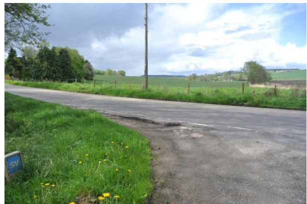
Minor access adjacent to B9161 south of Little Mill
