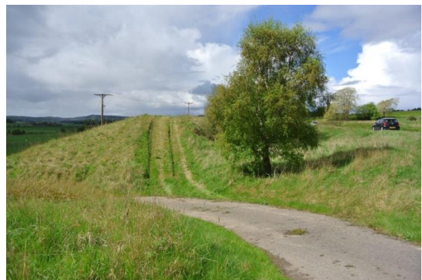
Disused rail line looking west
