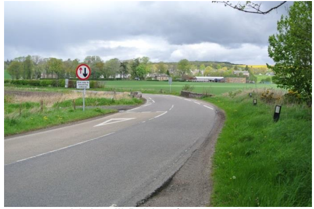
Littlemill Bridge from south
